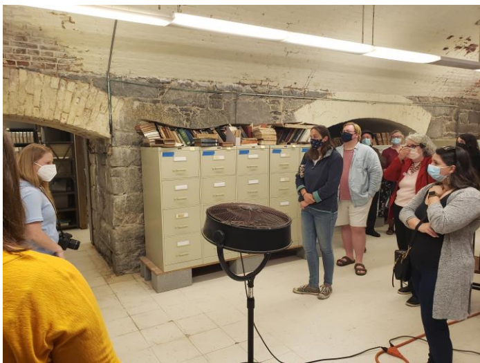
Fans are used to assist with air circulation in storage areas
