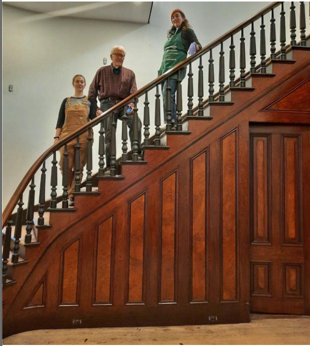
Original faux walnut- and burl-walnut-panelled staircase in the central hall, after cleaning, consolidation and inpainting (left to right Claire Martin, Carey Howlett, Talitha Daddona).
